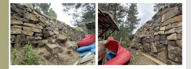
View looking north, this shows a section of the wall that has failed to the far east.
