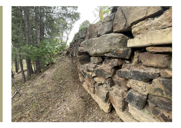
View looking west, this shows a section of the wall that has failed.
