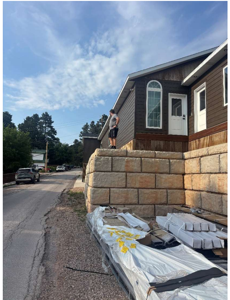
NEW CONSTRUCTION LOCATION FOR FRONT DECK REPLACEMENT
