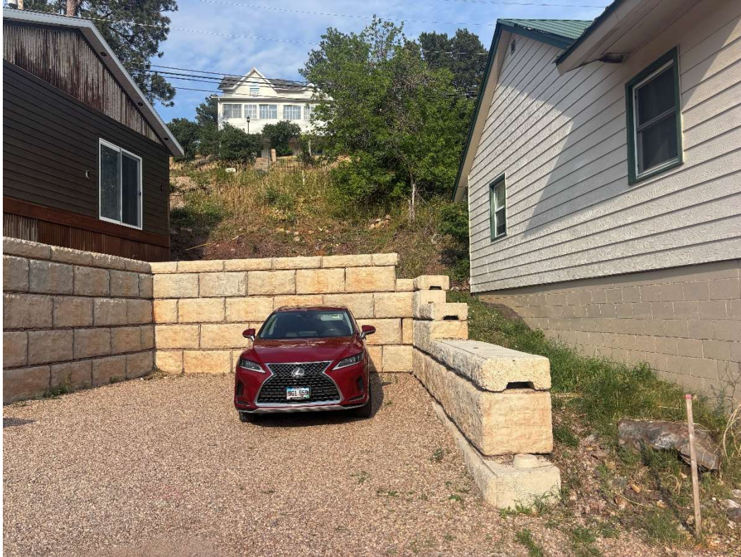
NEW CONSTRUCTION LOCATION FOR SIDE DECK REPLACEMENT
